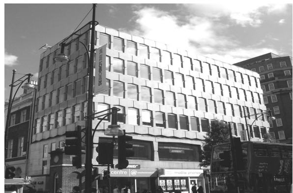
Figure 16: Nos. 354 - 358 Oxford Street
