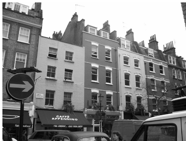
Figure 25: nos. 30 - 38 James Street (east)
