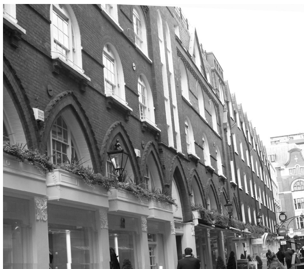
Figure 20: Nos. 23-31 St Christopher's Place
