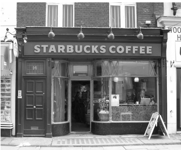
Figure 34: No. 14 James Street
