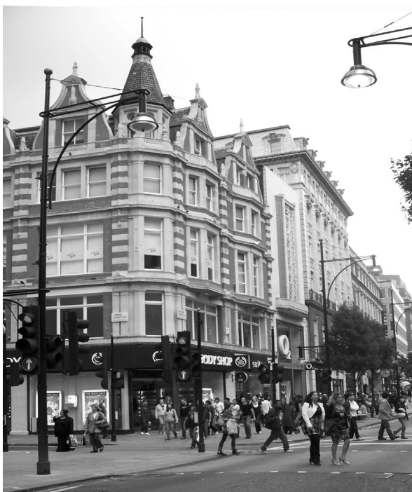
Figure 17: Nos 366 - 374 Oxford Street
