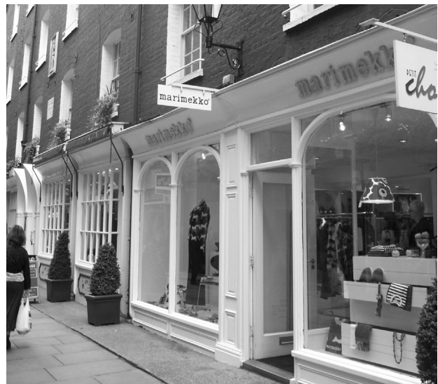
Figure 32: Shopfronts on St Christopher's Place
