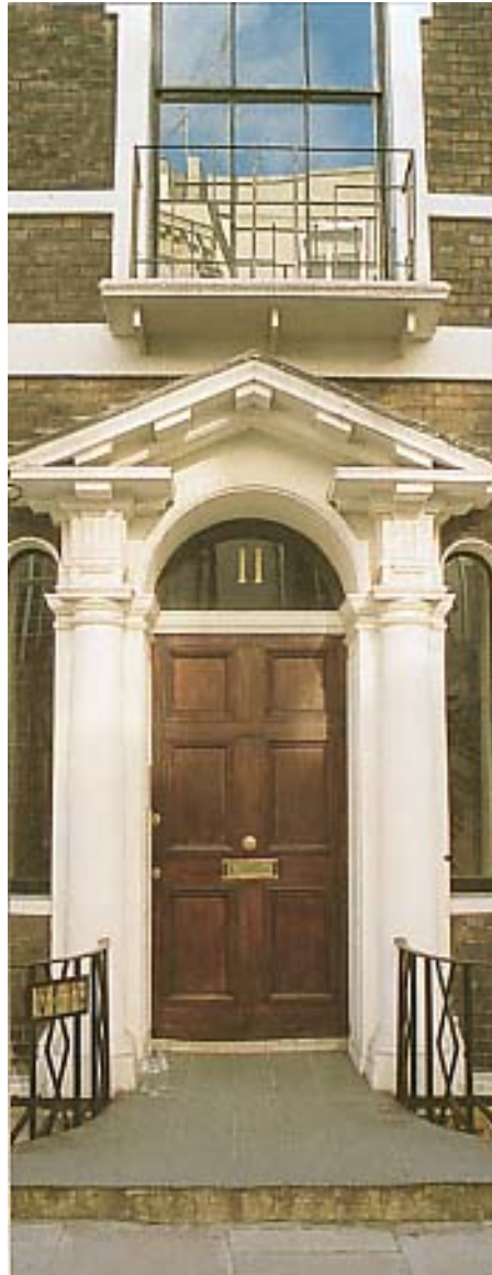
Entrance to 1760's townhouse. Wood doorcase of engaged Doric columns, panelled door and sidelights with fanlight over (11 Queen Anne Street, W1)
