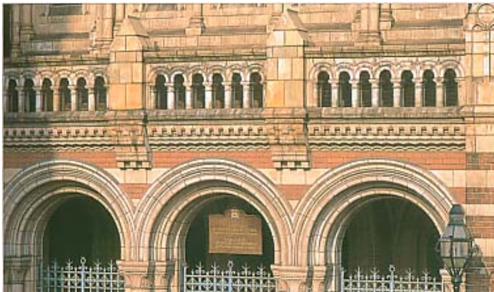
Terracotta façade produced by Burmantofts to designs by Alfred Waterhouse (1889-91). Ukrainian Catholic Cathedral, Duke Street, Mayfair, formerly King's Weigh House Chapel. Listed Grade II*.
