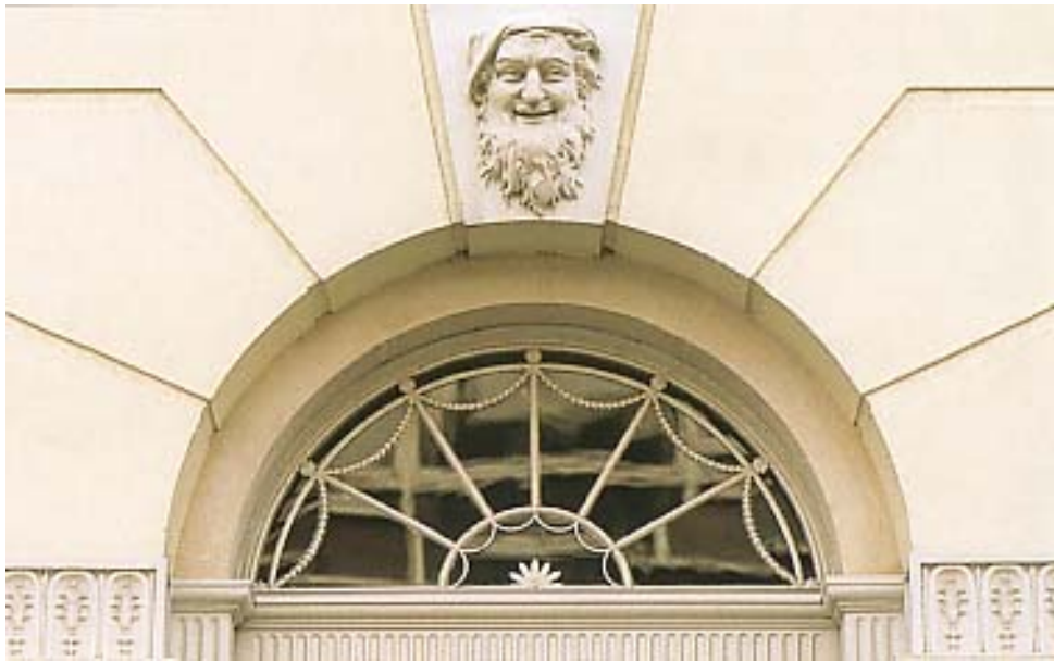
Manchester Street, W1. Stucco details around fanlight on a replicated façade.
