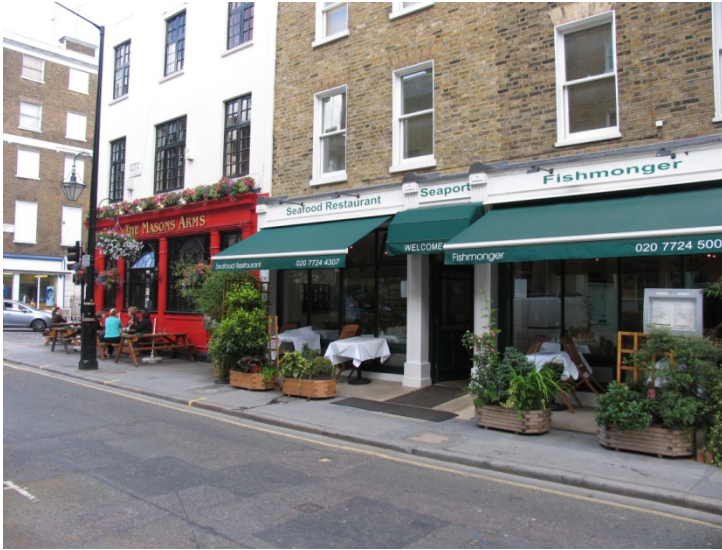
Attractive and well maintained shop fronts at the top of Seymour Place.
