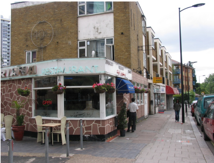
The Bourne Terrace frontage, with litter on the street, unattractive shop fronts and some vacant units.
