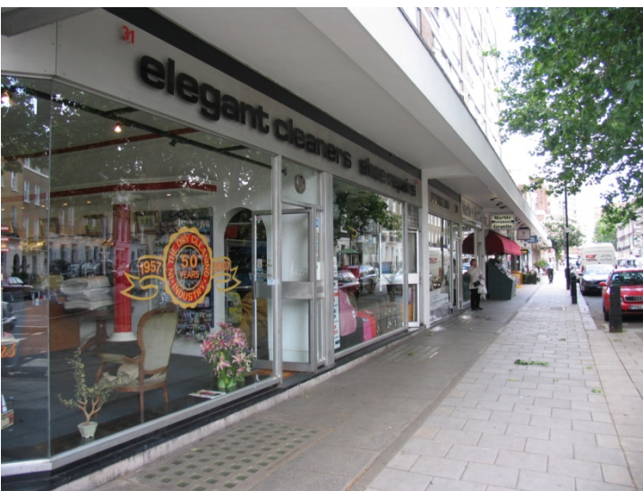
Purpose built covered shopping promenade at Coniston Court in the core shopping area.
