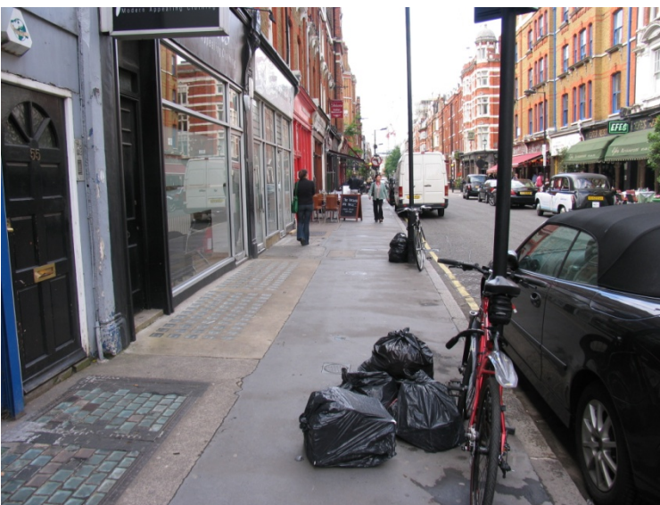
The west side of Great Titchfield Street, illustrating the narrow pavements in the centre, along with refuse left on the street and other clutter.
