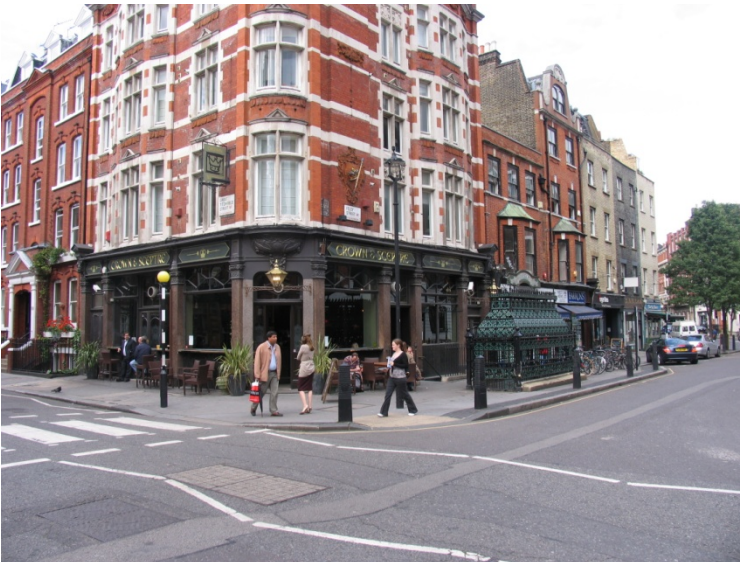
The northern part of the local centre with a reasonably attractive public house, which however contributes to street litter.
