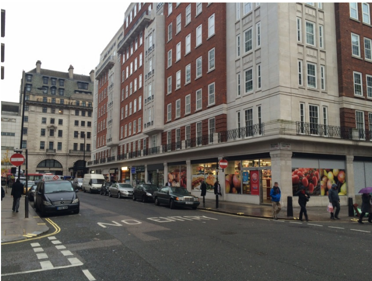
Busy pedestrian scene on Melcombe Street (looking back towards Baker Street).
