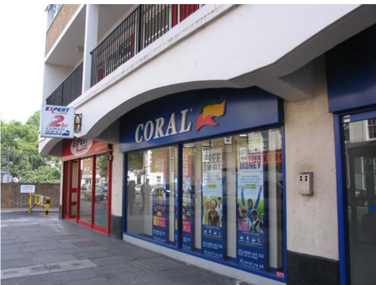
Another view of the secondary frontage on the south side of the local centre. A1 convenience (dry cleaner) and A2 use (betting office)
