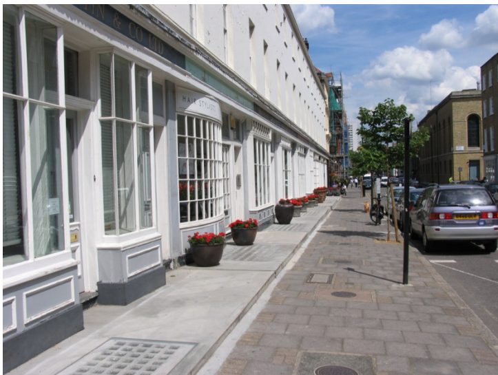
The attractive and well kept shop fronts and streetscape along York Street, at the north of the local centre.
