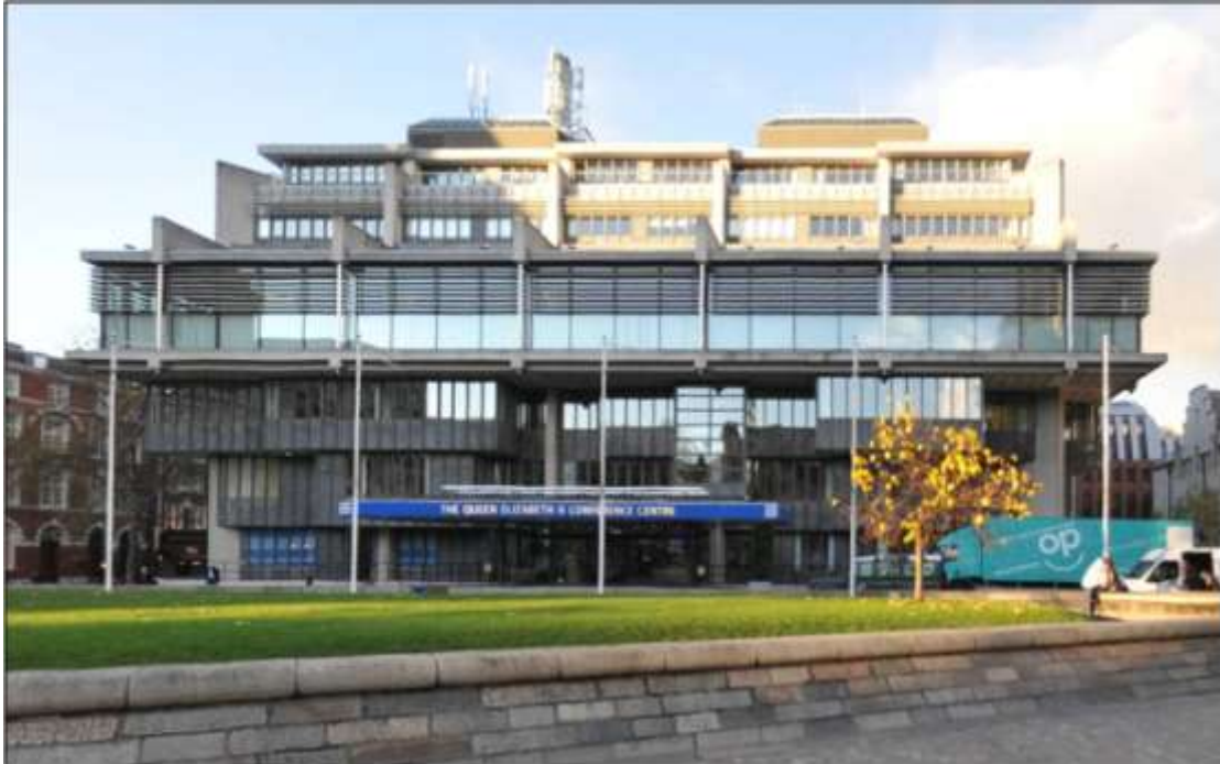
Figure 24: The Queen Elizabeth II Conference Centre as viewed from Victoria Street (Source: WCC iLookAbout January 2011).
