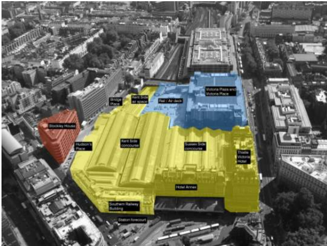
Figure 19: Victoria Station: Development is highly constrained by operational railway and listed building issues on the yellow shaded areas. The area's shaded blue are priorities for further change on the airdeck and inside the retail area above the platforms of the Victoria Plaza. The red shaded building is presently owned by a third party but could form part of an integrated development (source of main photograph from Network Rail)
