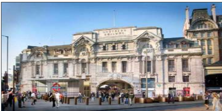
Figure 22: Victoria Station Upgrade
