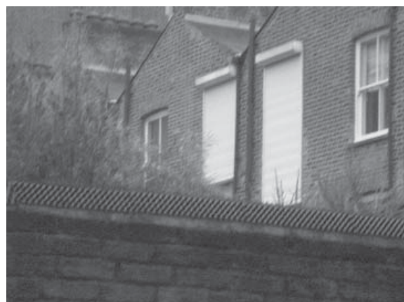
Figure 103: Roller shutters
