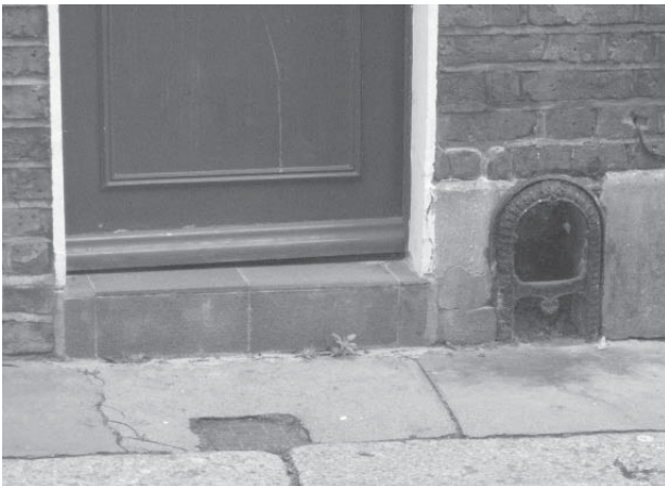
Figure 84: Bootscrape to No. 49 Greencoat Place
