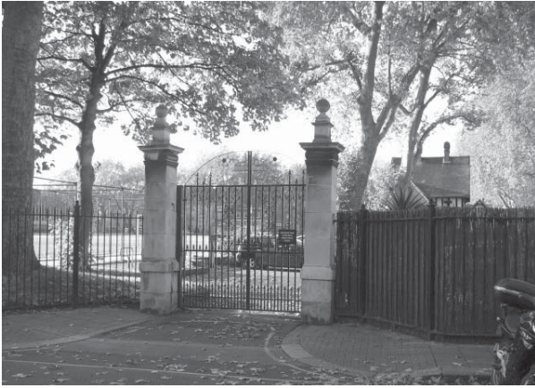
Figure 78: Stone gate piers to Vincent Square
