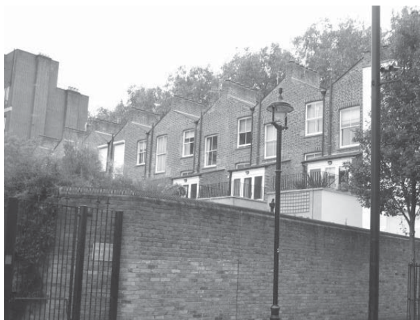
Figure 64: Rhythm of butterfly roofs maintained to the rear of nos. 37-45 Vincent Square
