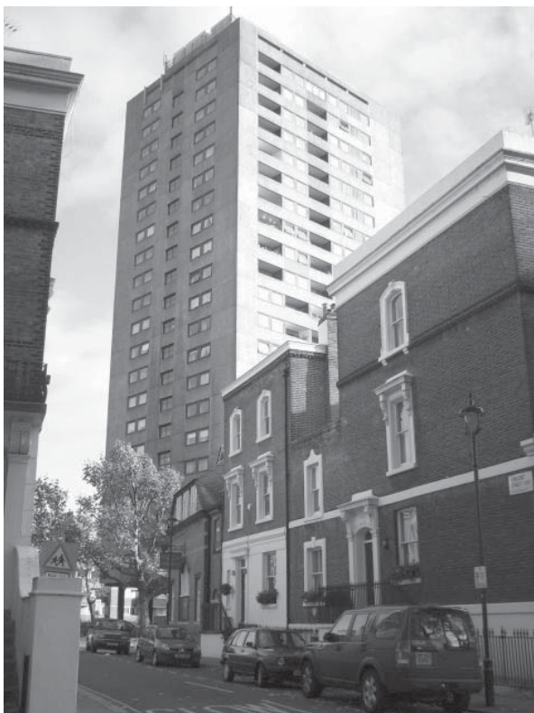
Figure 112: The Hide Tower has a significant impact on the character of the Vincent Square Conservation Area
