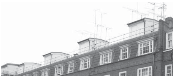
Figure 101: Roofscape to Carey Mansions, Rutherford Street
