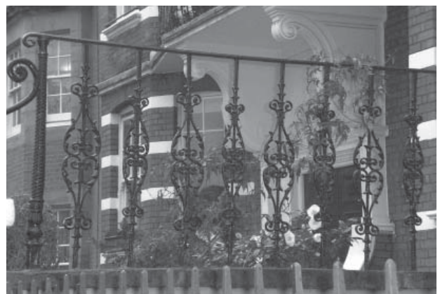
Figure 82: Delicate decorative side railing panel to The Willows.
