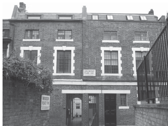
Figure 34: Nos. 55a and 55b Greencoat Place
