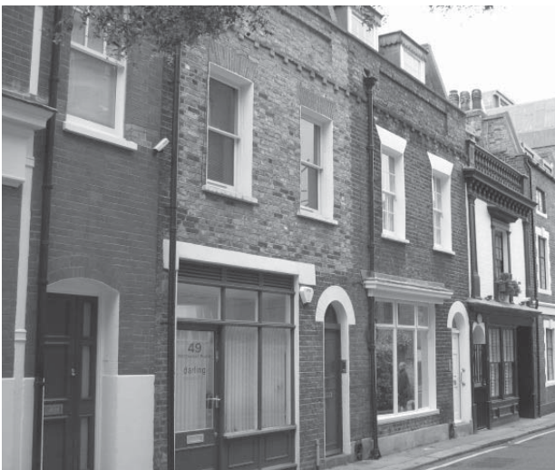
Figure 25: Nos. 49-51 Greencoat Place
