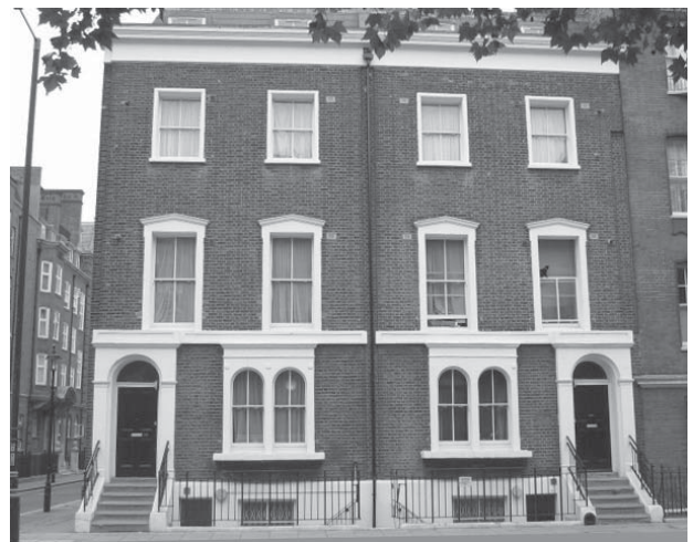
Figure 30: Nos. 144 and 146 Vauxhall Bridge Road
