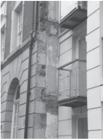
Figure 107: The exposed return elevation to no. 69 Rochester Row
