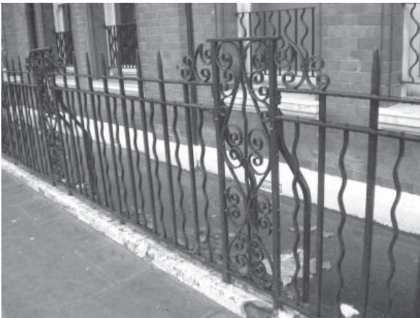
Figure 79: Railings to St Augustine's Mansions incorporating decorative scrolls and wave uprights
