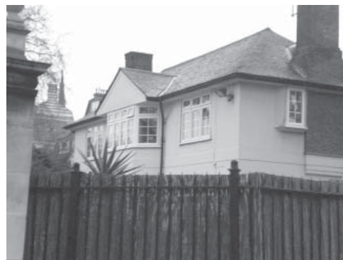
Figure 102: Replacement windows in uPVC
