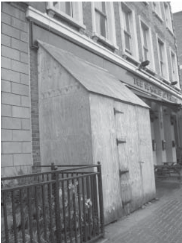
Figure 108: Temporary timber structure outside The Surprise at Pimlico Public House
