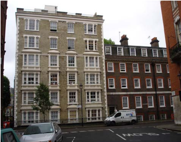
Figure 52: Improved Industrial dwellings flats and 29 Francis Street
