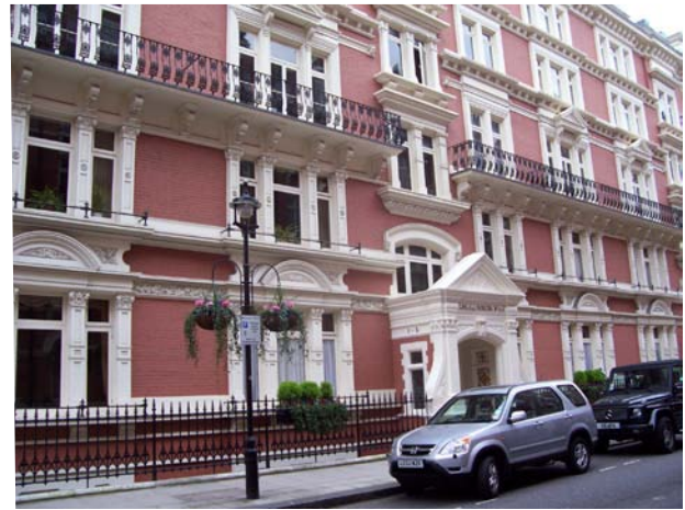
Figure 29: Nos 1-20 Carlisle Mansions, eastern facade of Carlisle Place
