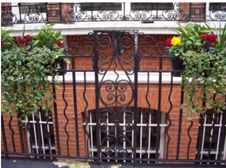
Figure 80: Victorian railings with delicate detailing on western Carlisle Mansions
