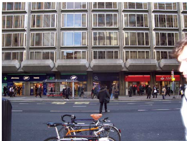
Figure 70: Ashdown House facade and shopfronts
