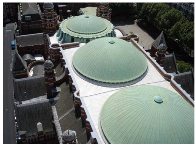
Figure 16: Aerial photo, Cathedral Roof
