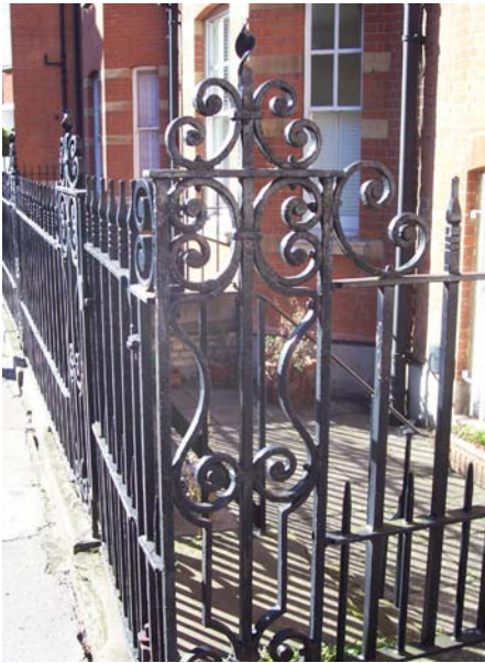
Figure 78: Early 20th century railings with wrought iron twisted leaves on corner of Emery Hill Street
