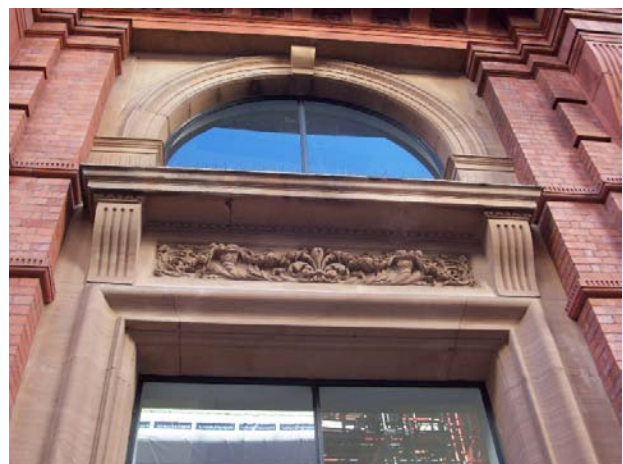
Figure 55: Greencoat House entrance
