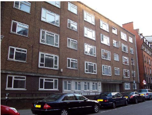
Figure 104: Victoria House, Francis Street
