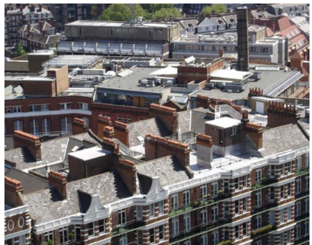
Figure 66: Ashley Garden Thirleby Road roofprofile showing pitched roofs with stout brick chimneys. Plant housings and lift overruns are incongruous features on the roofscape.
