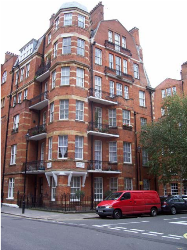
Figure 48: Nos. 216-227 Ashley Gardens, Emery Hill Street
