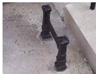
Figure 82: Original bootscrapers outside No. 1 Carlisle Place
