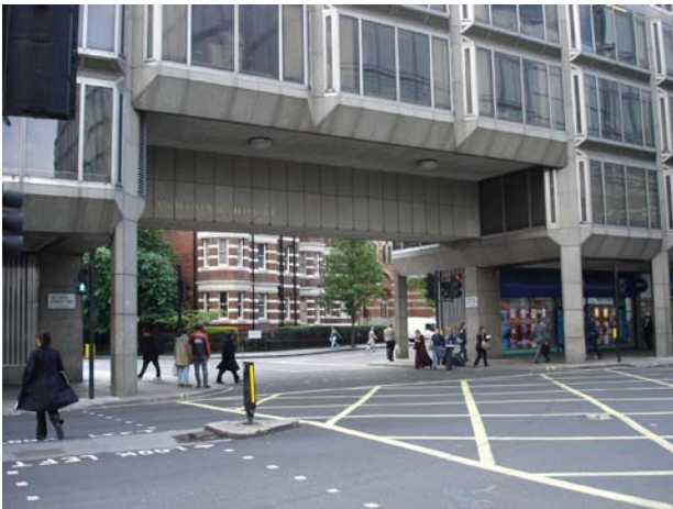
Figure 63: Ashdown House, archway to Thirleby Road
