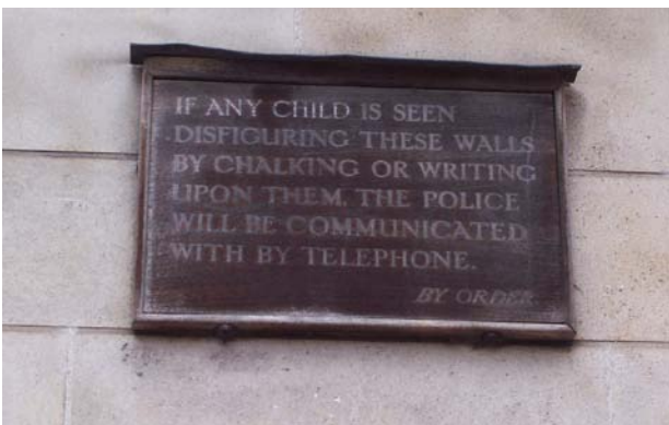
Figure 89: Wall mounted sign on Ambrosden Avenue side of Clergy House - "IF ANY CHILD IS SEEN DISFIGURING THESE WALLS BY CHALKING OR WRITING UPON THEM, THE POLICE WILL BE COMMUNICATED WITH BY TELEPHONE." BY ORDER
