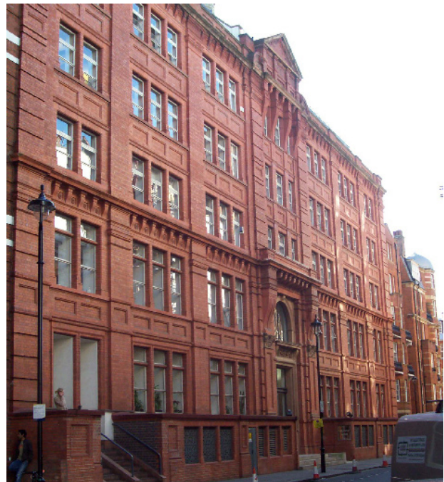
Figure 54: Greencoat House, converted offices
