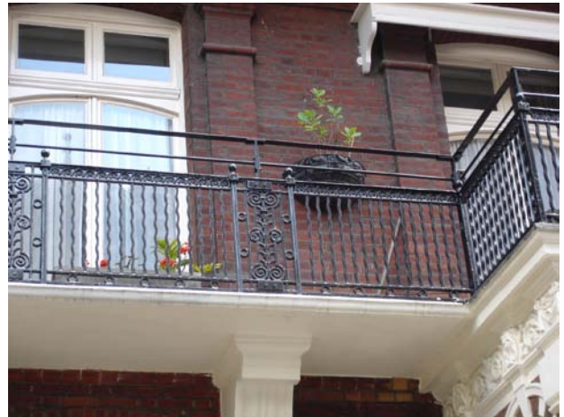
Figure 79: Balcony No.1-14 Ambrosden Avenue
