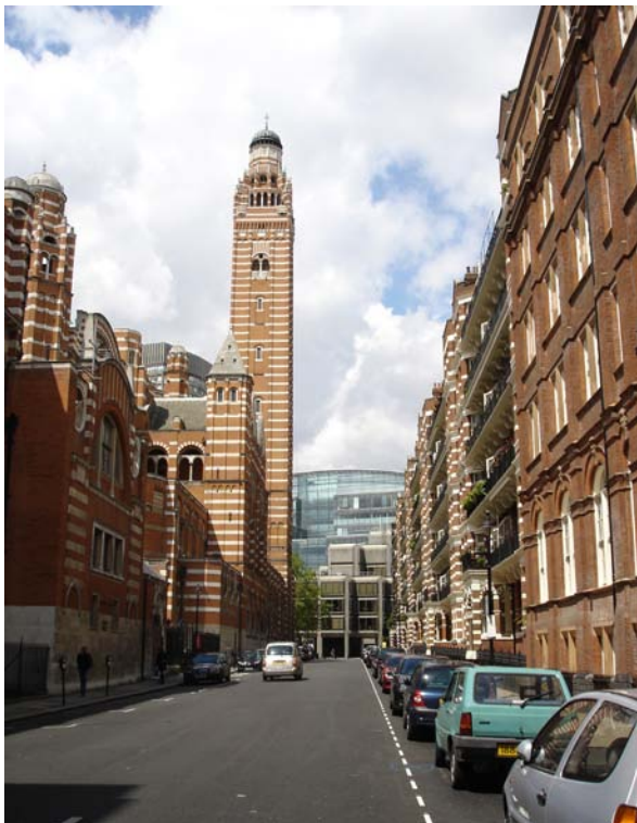
Figure 11: Ambrosden Avenue streetscape with cathedral to the left and mansion blocks on the right. The Cardinal Place development on Victoria Street can be glimpsed.
