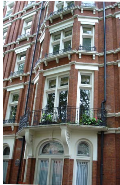
Figure 37: Bay windows. Nos 1-24 Morpeth Mansions
