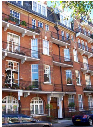
Figure 50: No.182-186a Ashley Gardens, front facade
