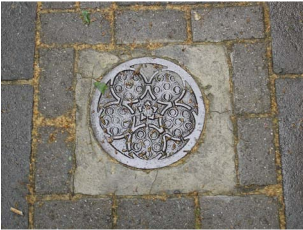
Figure 95: Coal Hole Cover. Morpeth Terrace
