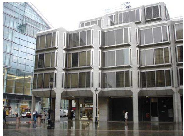
Figure 62: Ashdown House, piazza facade
