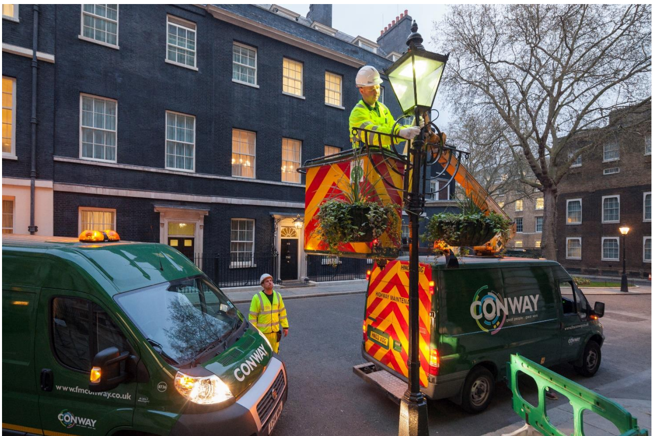
Maintenance operations Downing Street
