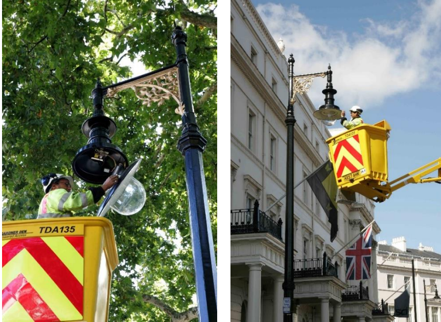
Public lighting maintenance operations
