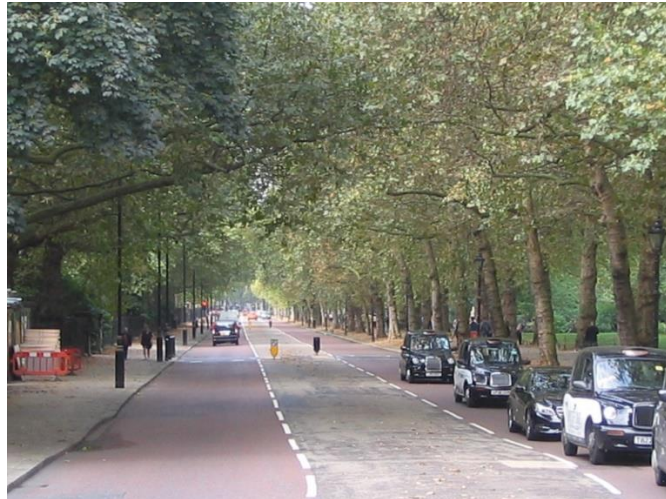
Birdcage Walk, the lighting on the right hand side (path lighting) is of a height where it sits below the tree canopies, however the lighting on the left (road lighting) being higher is now within the tree canopies, affecting the performance of the installation and communication of the control system.
