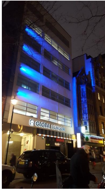
Poor lighting design with excessive spill light
