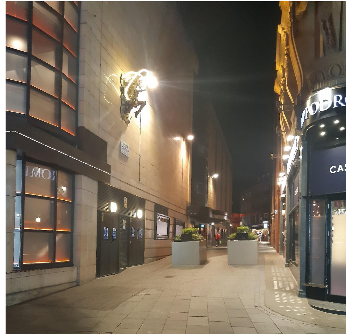
Image 25: Wall mounted installation Leicester Court
