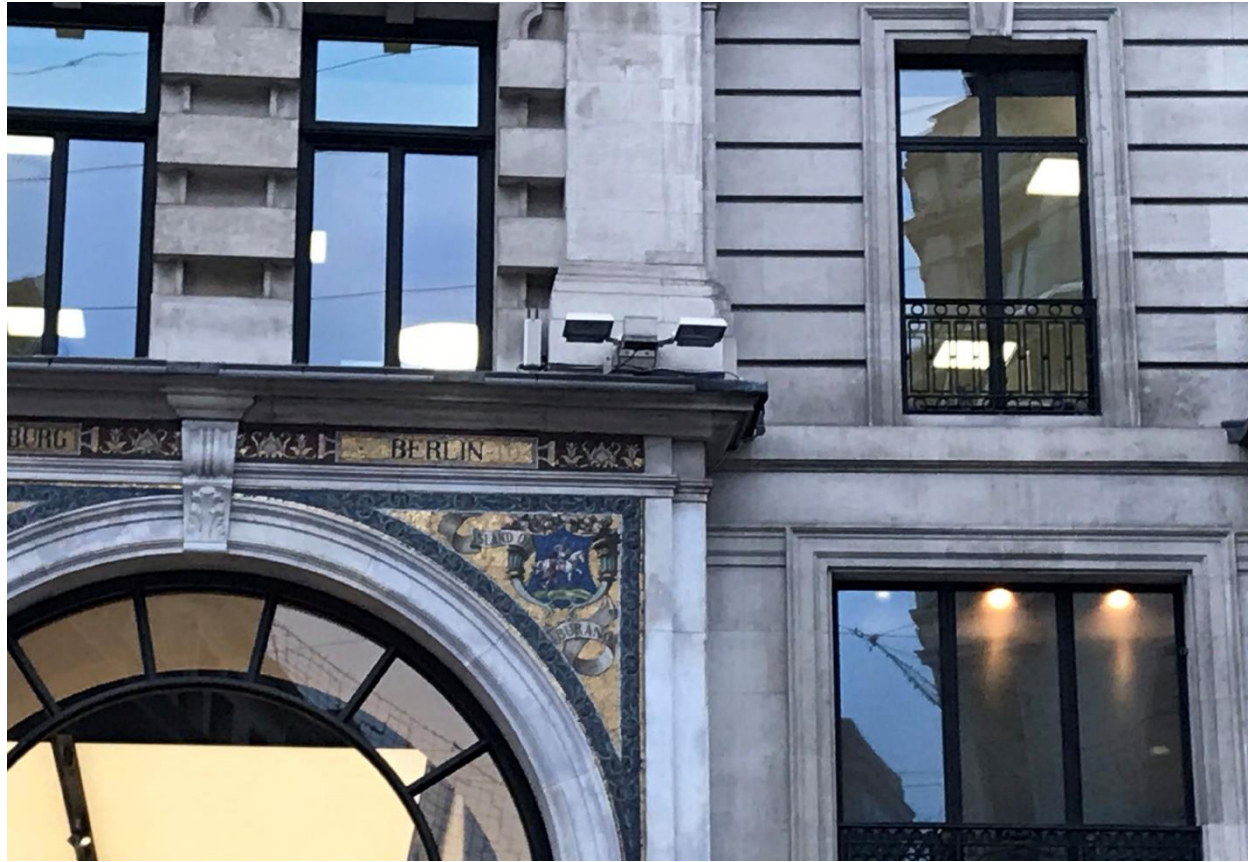
Image 26: Wall mounted installation- Regents Street
