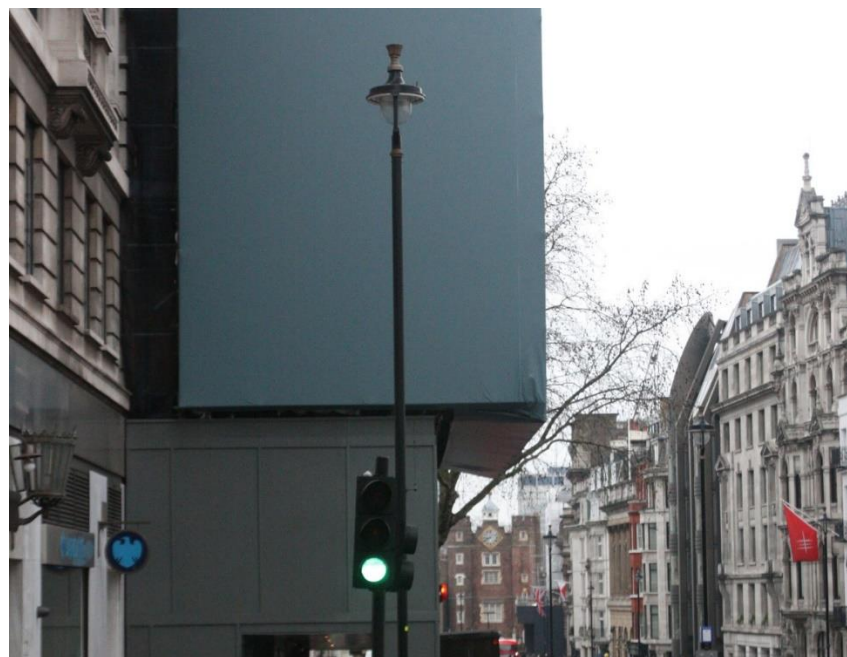
Image 53: Hoarding affecting the performance of column lighting
