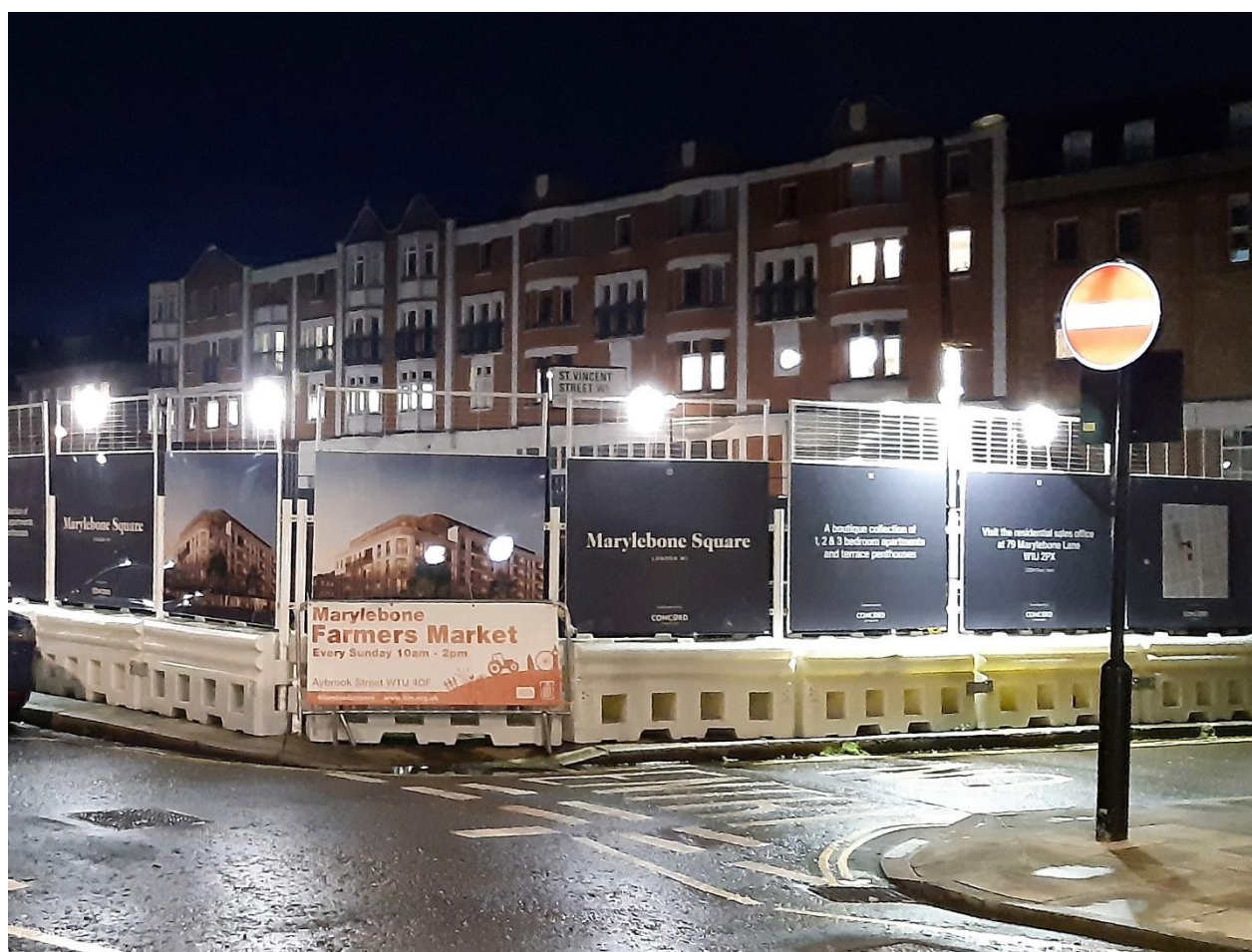
Image 57: Example of good hoarding lighting
