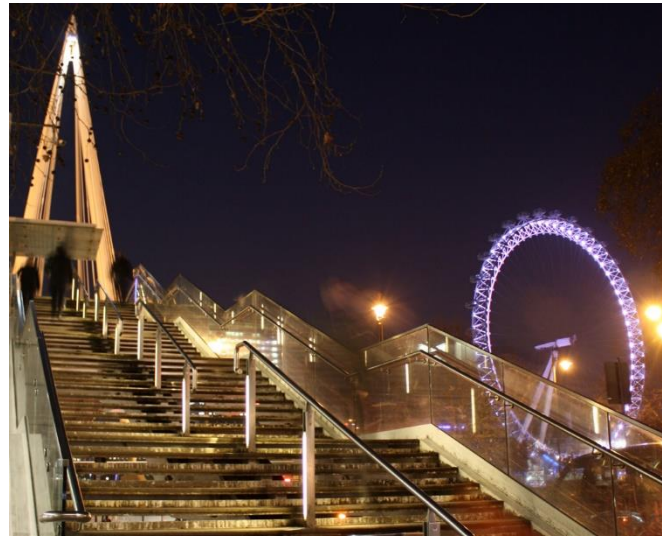
Image 2: Stairs, Golden Jubilee Footbridge
