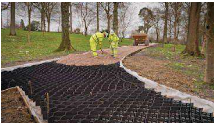
Figure 18: Indicative Cellweb Installation
