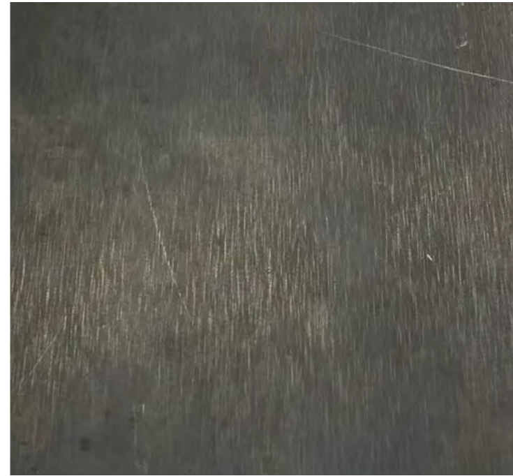
Blackened steel - doors to courtyard
