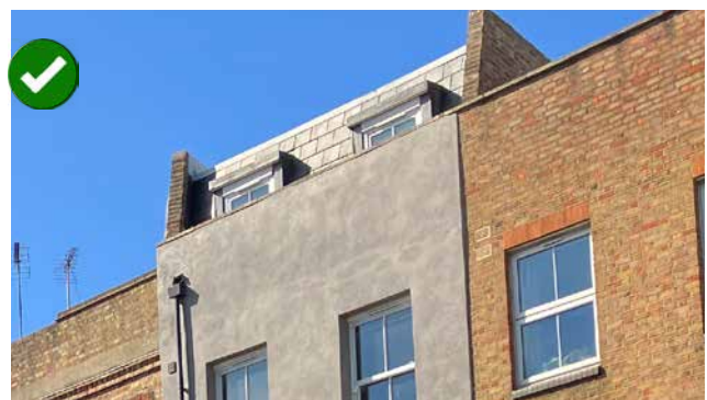
Figure 70: Diagram showing dormers that are obscured behind the parapet wall from the street below, Maida Hill
