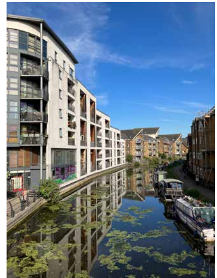
Figure 45: View from Half Penny Steps footbridge
