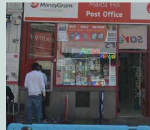
Large shop window with timber frame
