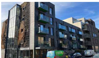
New residential building in Fermoy Rd,
