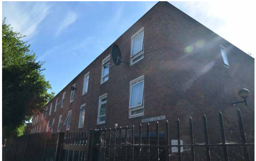
Figure 29: Terraced housing with black metal railings as boundary treatment, Fernhead Road
