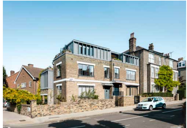
Figure 75: 32 Laurier Road - extra floor added to facilitate family living. Richard Keep Architects (photo credit: Ben Blossom).
