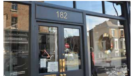
Large glazed shop front windows
