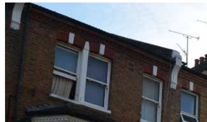
Double hung sash windows
