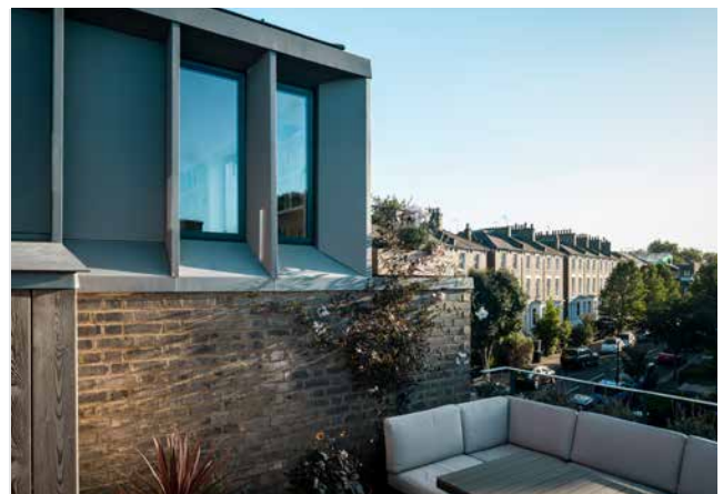
Figure 77: 32 Laurier Road - extension with roof terraces settling into the Victorian character of the street. Richard Keep Architects (photo credit: Ben Blossom).
