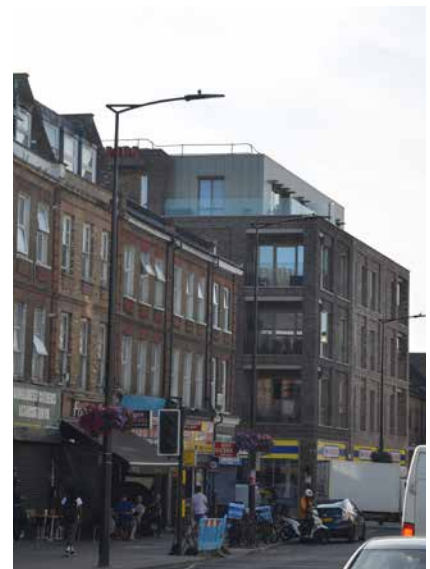
Figure 37: Elgin Estate redevelopment
