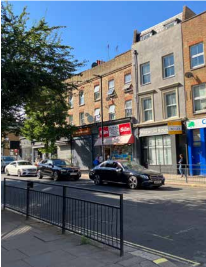
Figure 23: Ground floor retail buildings with housing above, Shirland Road
