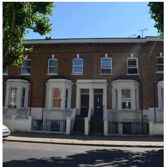
Figure 62: Example of dormer property with a roof extension and dormer windows
