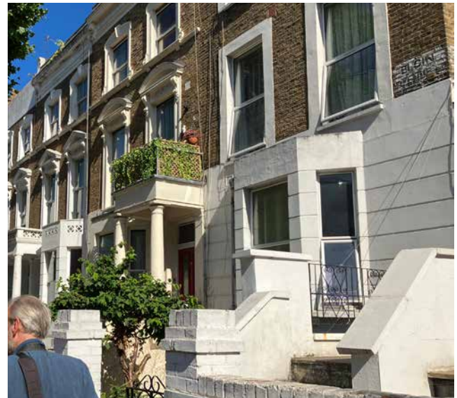
Figure 33: Typical Victorian architectural frontage in the character area, Elgin Avenue
