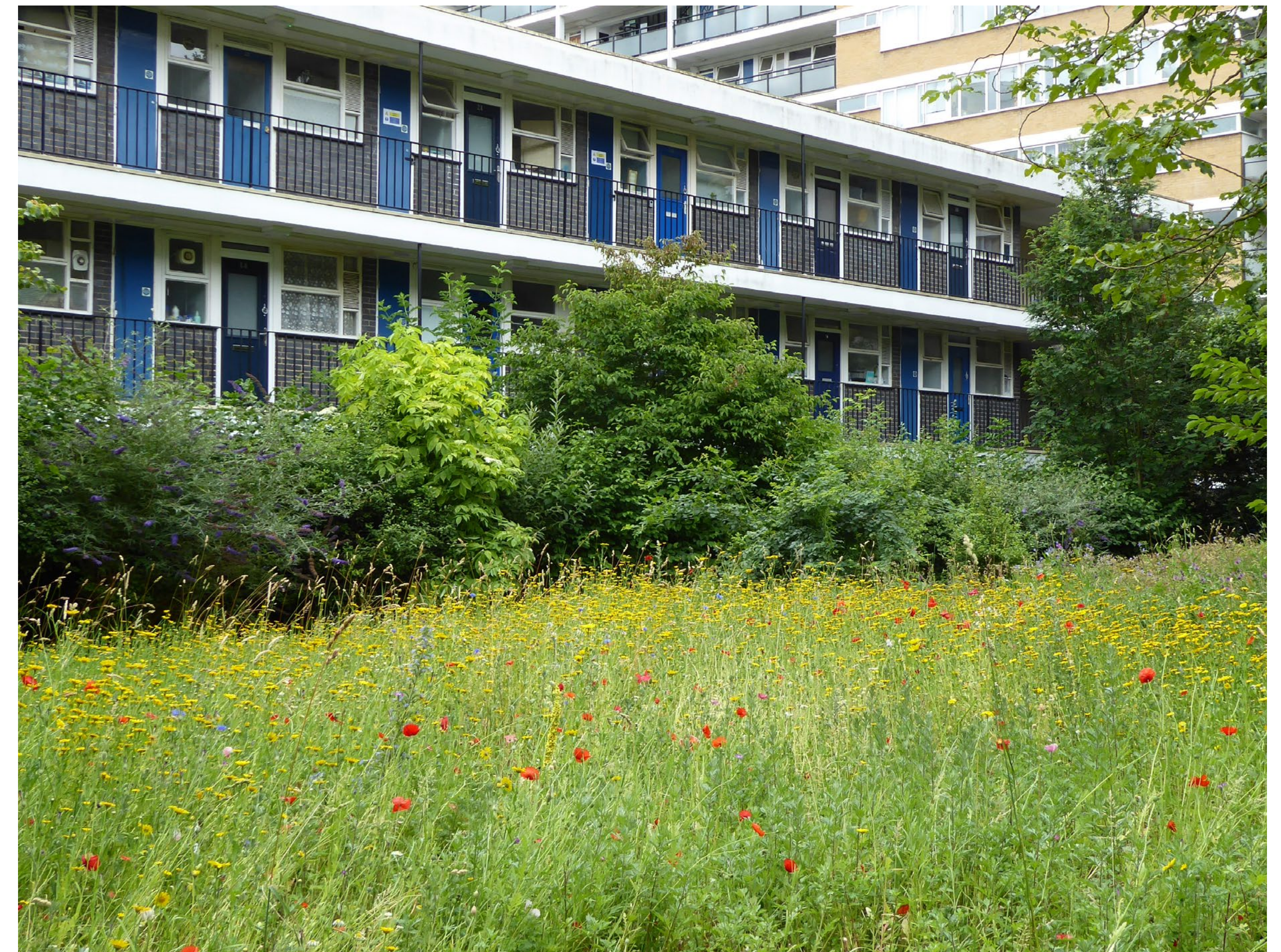
Greening on Churchill Gardens housing estate
