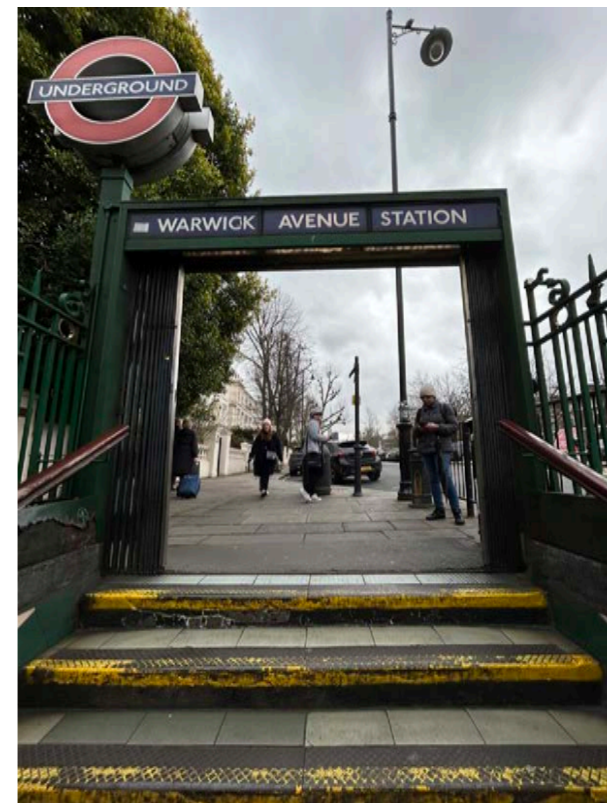
“The station stairs are an accident waiting to happen.”
