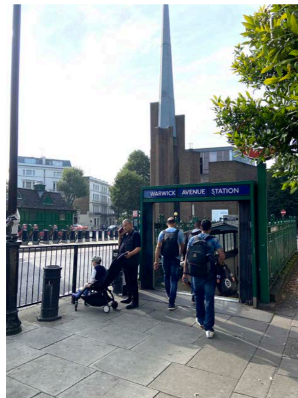
“The Tube entrance is disgusting. The tiles are broken, the planting isn’t working, it’s dark and it’s like going into a bomb shelter.”
