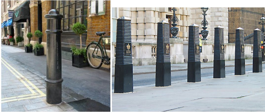
Figure 38: Example of Cannon Heritage cast iron bollard in Westminster.
