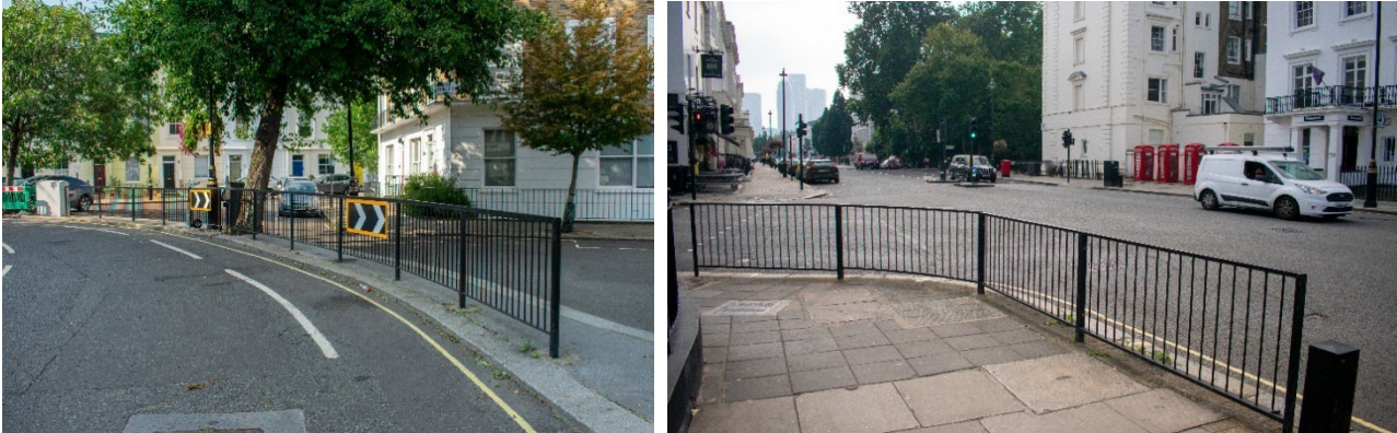
Figure 40: Examples of guardrails in Westminster.
