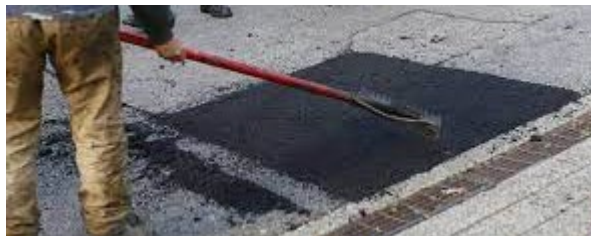
Figure 61: Example of repair works to surface damage.
