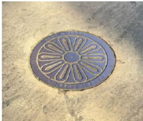
Figure 58: Example of Cast Iron Coal Hole cover.
