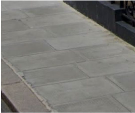
Figure 57: Example of concrete paving.
