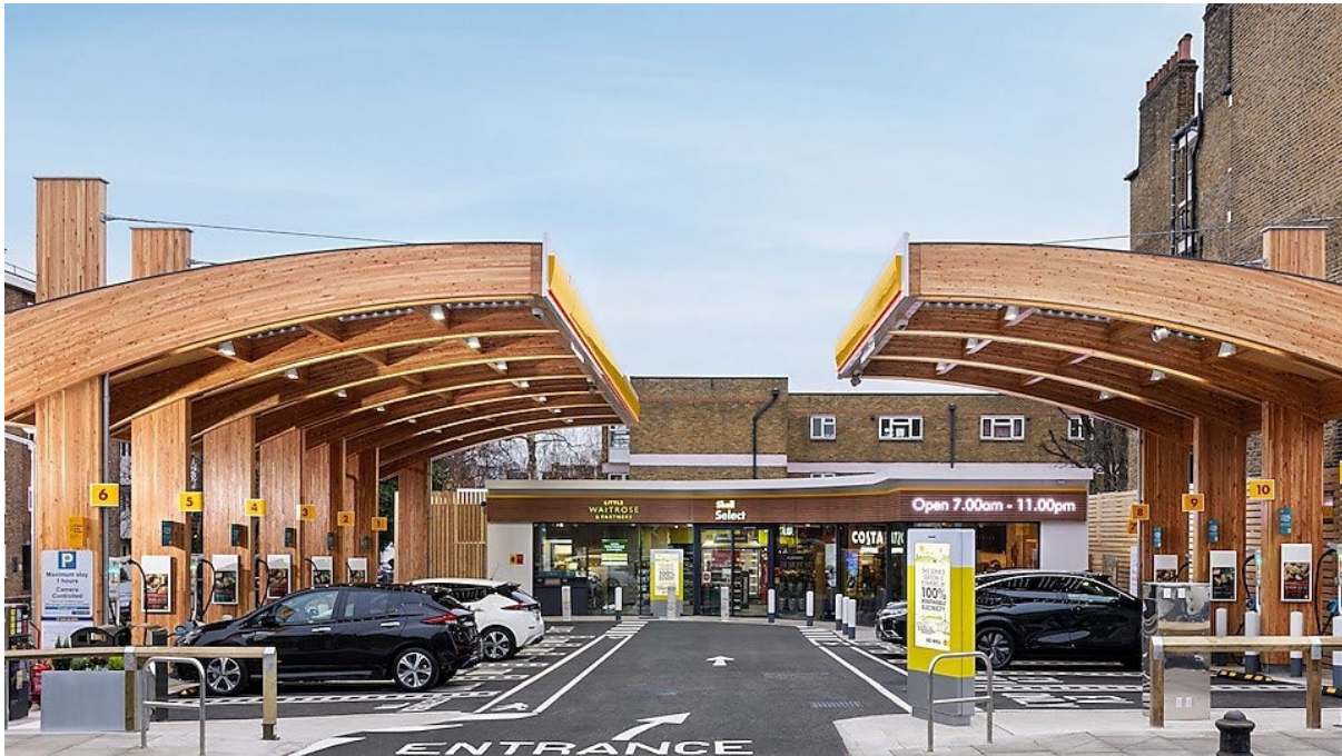
Figure 49: Example of Shell recharge station on Fulham Road.
